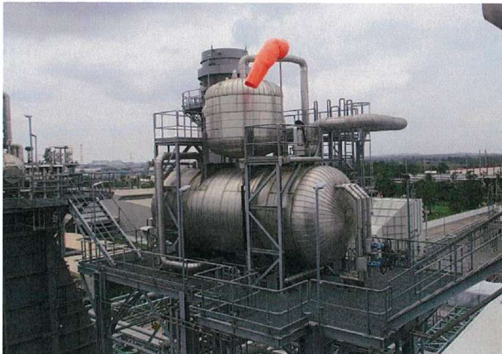
Feed Water Tank and Deaerator Drum
